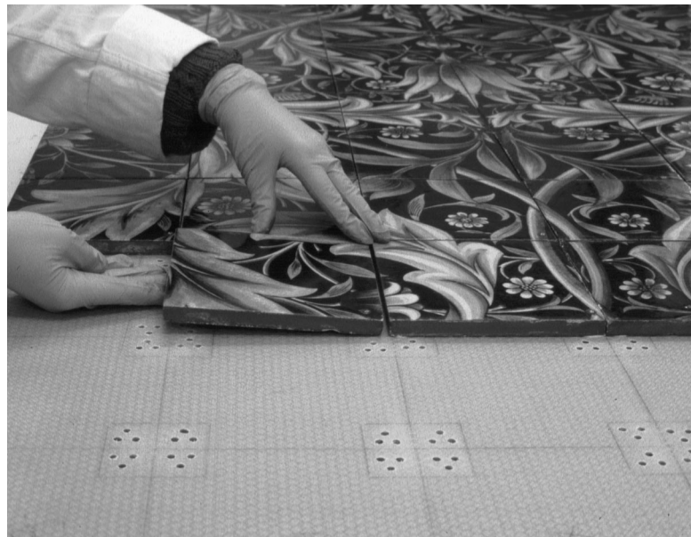
Figure 3 Mounting the tiles on a prepared Aerolam® board, photography Fiona Jordan
