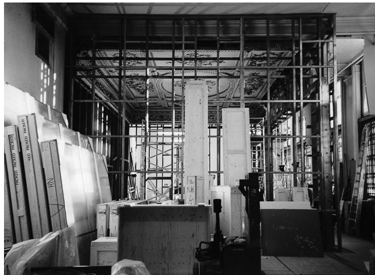
Figure 1: Dismantling of a period room in the British Galleries. Photo: Julie Taylor
