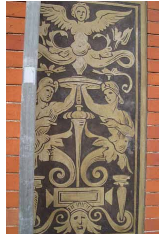
Detail from the newly consolidated sgraffito façade. A fresco style technique was used to re-establish the weathered decoration and protect the original sgraffito underneath
